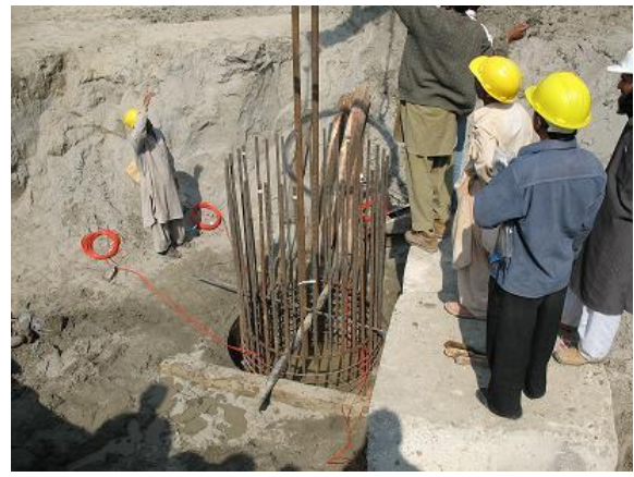
Above Left : The bottom section of the reinforcement cage is lowered into the borehole.
