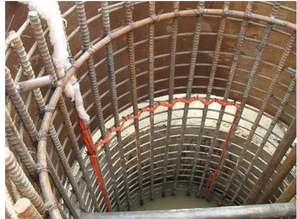
Above Left : Another task the technicians carry out as they climb the secured structure is joining the Extensometer tubes that run to varying depths inside the reinforcement cage. Once this is complete and the cabling is fastened the complete reinforcement cage is lowered to the full depth.
