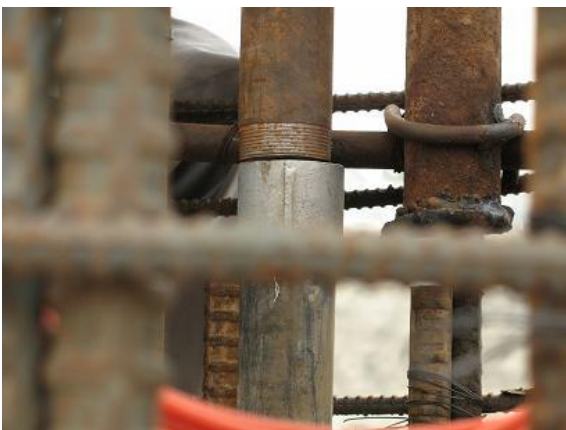
Above Left : Another task the technicians carry out as they climb the secured structure is joining the Extensometer tubes that run to varying depths inside the reinforcement cage. Once this is complete and the cabling is fastened the complete reinforcement cage is lowered to the full depth.
