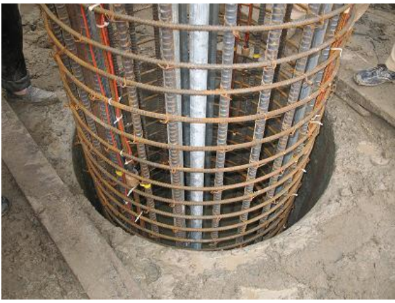
Above Left : The bottom section of the reinforcement cage is lowered into the borehole.
