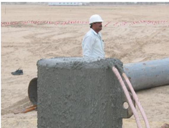
Above Left: The pile as observed after the concreting is finished, the final part of the process is to remove the casing from the top ready for the construction of the top cap.
