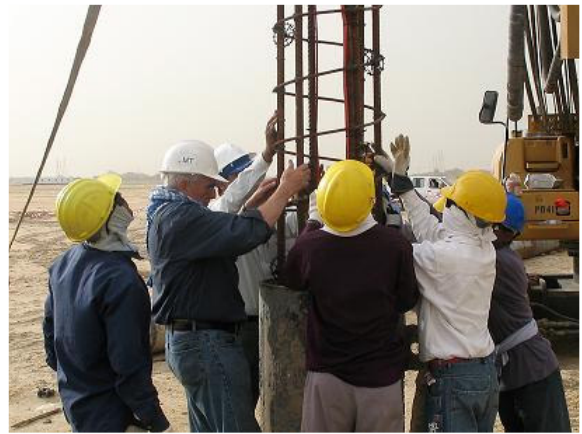
Above Left: The fully reinforcement instrumented cage ready to be lifted into the borehole. Visible at the top of the reinforcement cage are the sensor cables that have been wrapped in a protective plastic covering to ensure they do not come into contact with the concrete.
