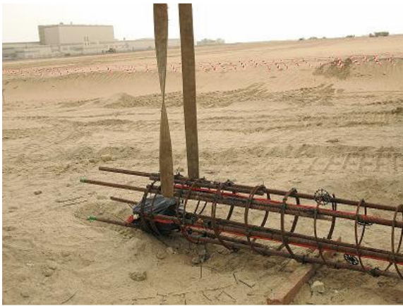
Above Left: The fully reinforcement instrumented cage ready to be lifted into the borehole. Visible at the top of the reinforcement cage are the sensor cables that have been wrapped in a protective plastic covering to ensure they do not come into contact with the concrete.
