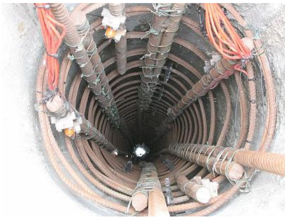
Above Left: A top down view of the pile cage resting in the borehole with the top layer of gauges clearly visible.
